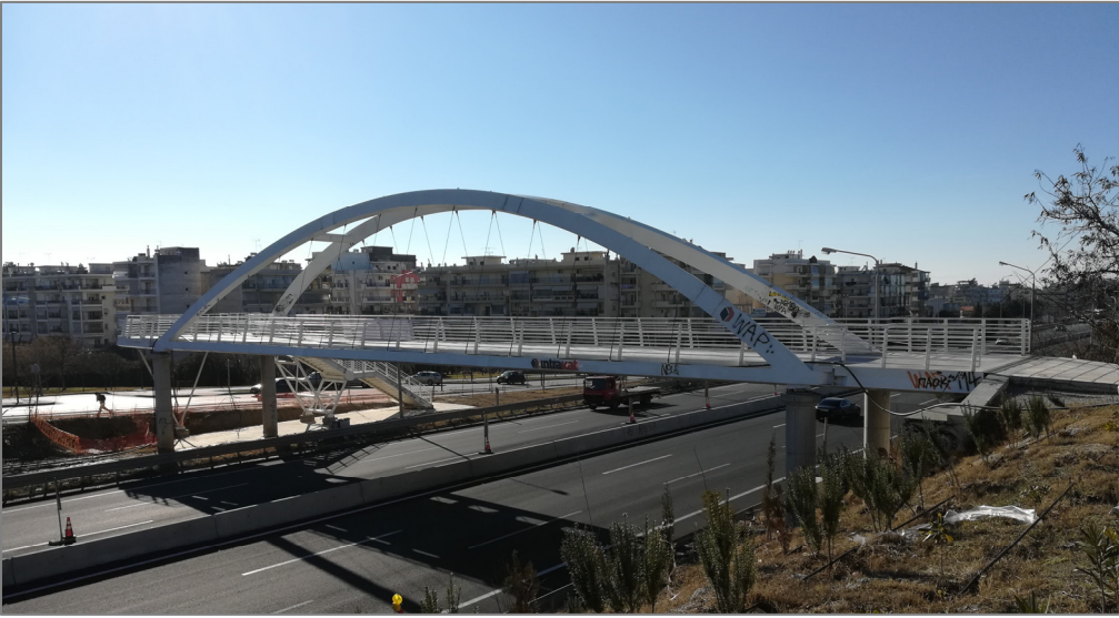
Figure 5: The pedestrian bridge in Evosmos, Thessaloniki, Greece
